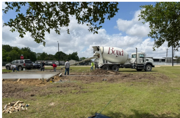
Boyd Ready Mix Donating Concrete
